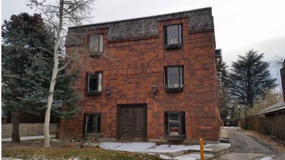
Multi-story flat roof building with less than 50% glazing.
